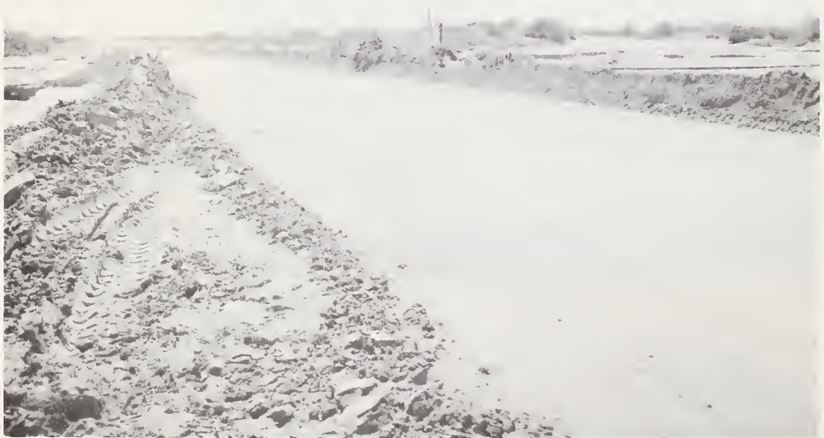
Highway 54 road damage Note sediment deposition.
